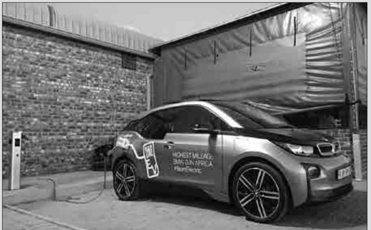
During last week an electric vehicle charger was installed at Buffalo Valley Spur in Heilbron. The Heilbron charger is part of the route to Clarens and part of the #evCrowdRoute planned rollout to make tourists visit towns they would ordinarily drive past. Over the next 10 years the company plans to install 11777 chargers, one for every town in South Africa.
